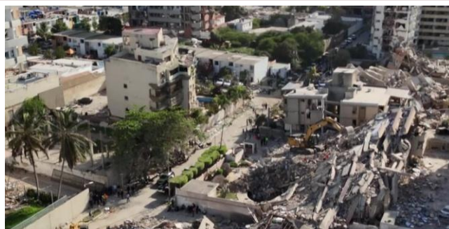
Aerial view of collapsed multi-story buildings and ground operations.
