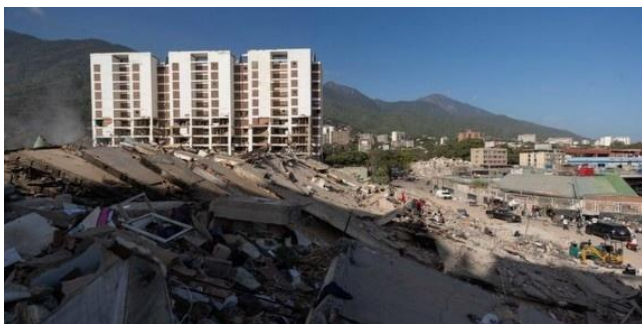
Panoramic view of structural collapse across the affected urban areas.
