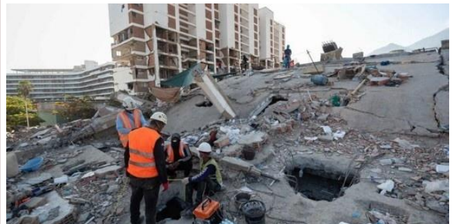
Rescue teams and volunteers conducting search operations in collapsed structures.
