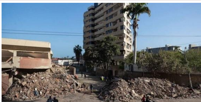
Severe structural damage to high-rise residential buildings.
